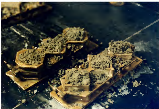
Figure 12. Filling the Molds. After mixing, the mortar was placed into the molds with a hand trowel. Overfilling of the molds was necessary to reduce the voids when tamped.
