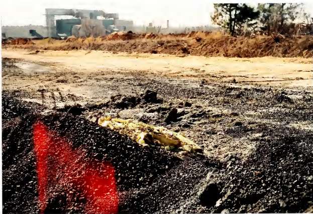
Figure 18. Waste sulfur, from the plant's sulfur injection system, is disposed of in the pond. The sulfur, sulfite ( \text{SO}_3 ), is injected into the exhaust gases to increase the effectiveness of electrostatic precipitators. The change to a low-sulfur coal about ten years ago forced GPC to use this system to comply with the standards for particulate emission within the Clean Air Act. Waste sulfur is generated usually during delivery when some will spill on the ground and is cleaned up and deposited in the pond.
